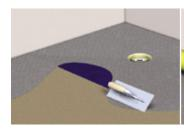
Apply tile adhesive to your floor former or floor substrate using a small notched trowel.
